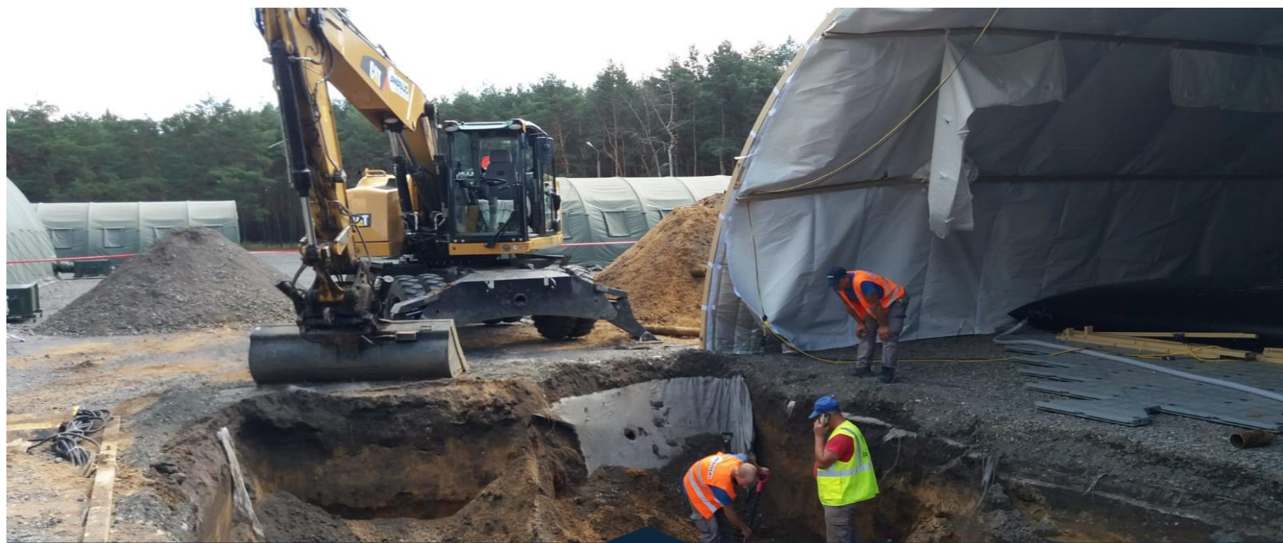
LSA GROUND WORKS
